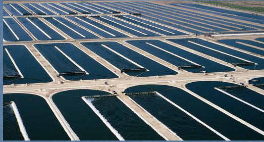
Open raceway paddle wheel mixed ponds now used by 98% commercial microalgae production. Products are pharmaceuticals not fuels. From J. R. Breneman at NREL-AFOSR Workshop, Arlington VA (2008).
